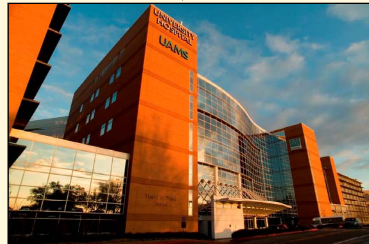
University Hospital Little Rock, Arkansas
