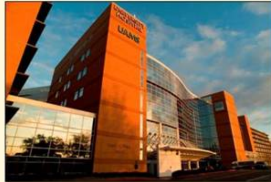
University Hospital Little Rock, Arkansas
